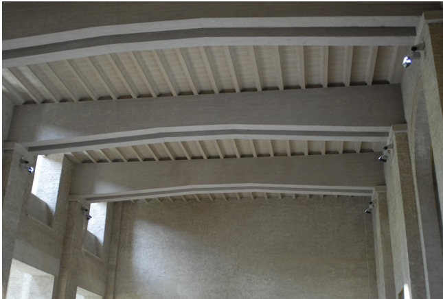
Figure 9: Entry vestibule, Alte Pinakothek. Katzenbach concrete beams in the vestibule ceiling. Photo by author
